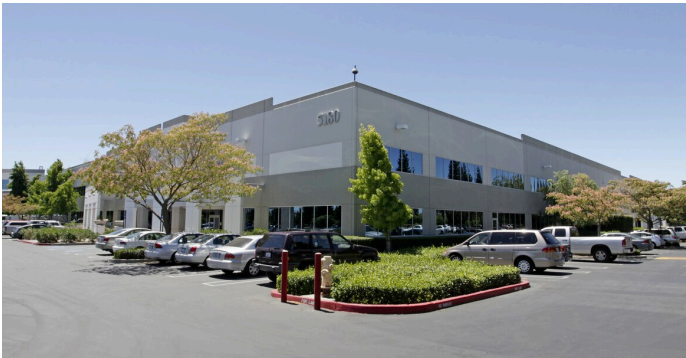
5160 Hacienda Drive, Dublin | 200,000 square feet
